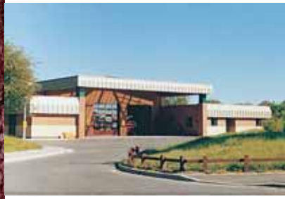
Bartley Green Fire Station
