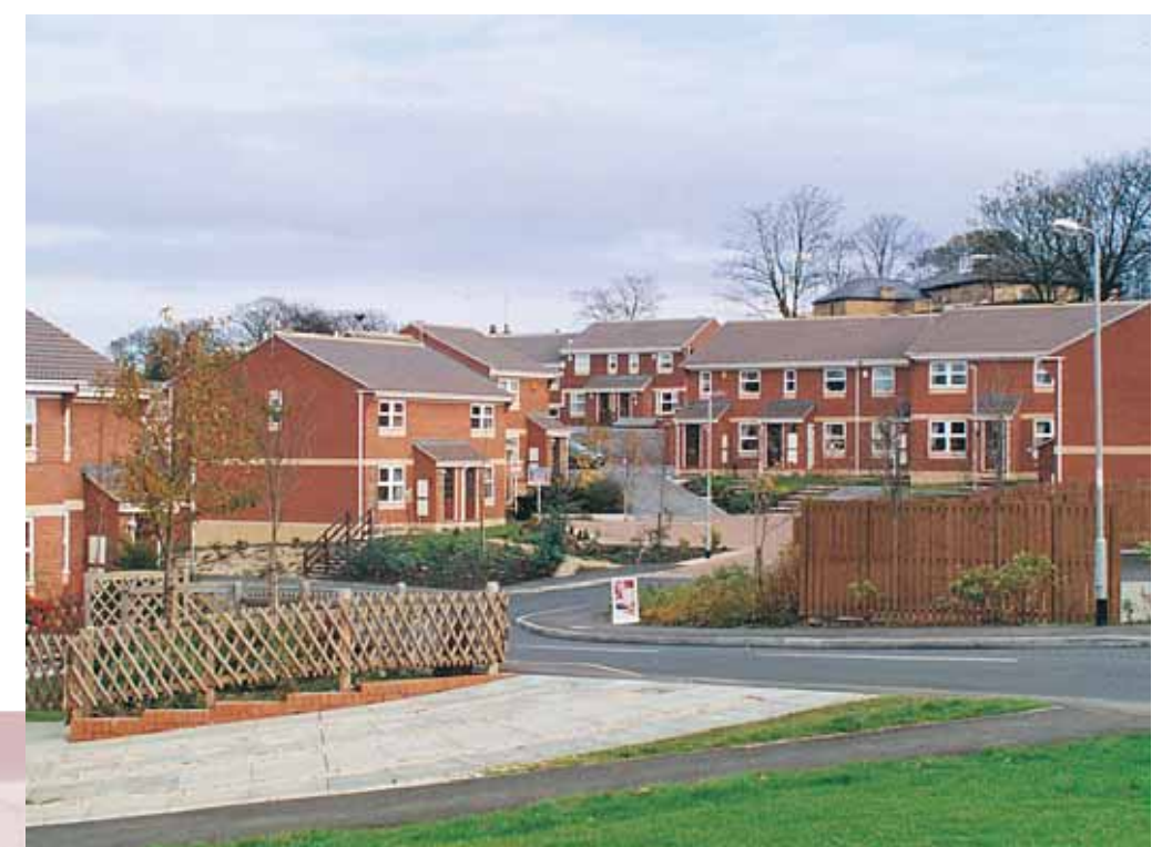
Barrett Homes, Leeds
