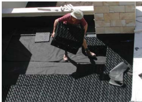
Installing tank modules into planter box
